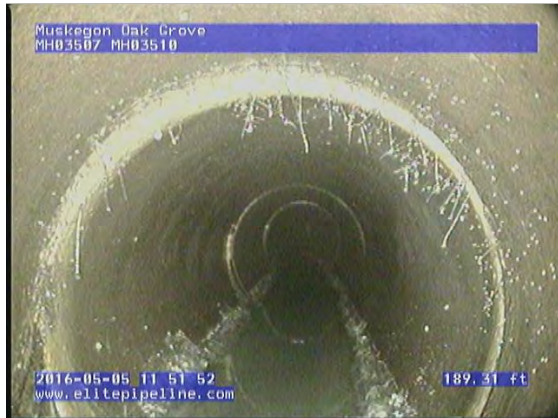
GM3676_29b5a4f6-782c-44a4-b604-e6dda5d2d56c_20160505_115329_603.jpg, 00:26:21, 189.31 Joint Offset Medium
