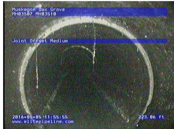
GM3676_29b5a4f6-782c-44a4-b604-e6dda5d2d56c_20160505_115732_073.jpg, 00:29:48, 223.06 Joint Offset Medium
