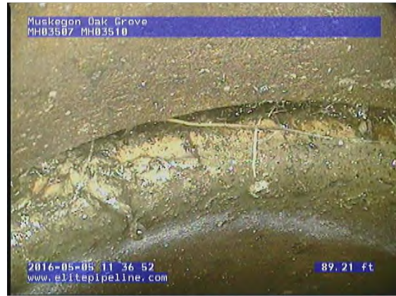
GM3676_29b5a4f6-782c-44a4-b604-e6dda5d2d56c_20160505_113829_023.jpg, 00:13:11, 87.89 Joint Offset Medium
