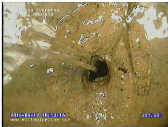
GM3702_bffedebf-8262-4dd8-8638-19abd94e99a5_20160512_101334_973.jpg, 00:18:31, 221.43 Hole at 11 o'clock
