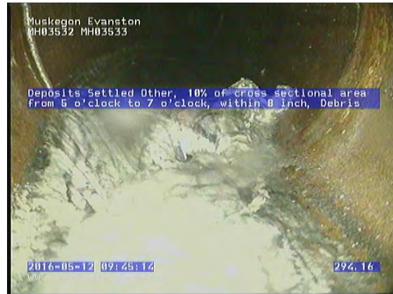
GM3701_62c62d3f-fa26-4182-aa9d-10e119c32db3_20160512_094633_088.jpg, 00:21:01, 294.13 Deposits Settled Other, 10% of cross sectional area from 5 o'clock to 7 o'clock, within 8 inch, Debris
