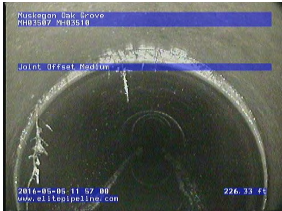
GM3676_29b5a4f6-782c-44a4-b604-e6dda5d2d56c_20160505_115836_850.jpg, 00:30:36, 226.32 Joint Offset Medium
