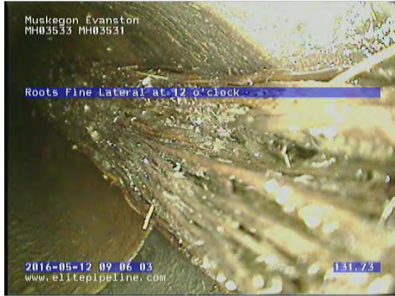
GM3700_d760bc2d-7738-420b-a21c-0e3d9fae79d8_20160512_090722_583.jpg, 00:09:39, 131.72 Roots Fine Lateral at 12 o'clock
