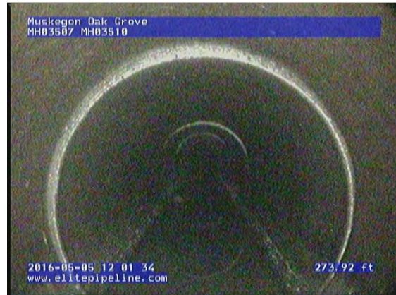
GM3676_29b5a4f6-782c-44a4-b604-e6dda5d2d56c_20160505_120311_463.jpg, 00:34:46, 273.92 Joint Offset Medium
