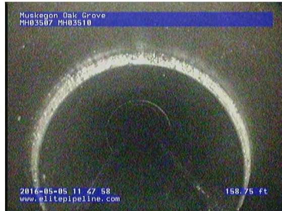
GM3676_29b5a4f6-782c-44a4-b604-e6dda5d2d56c_20160505_114935_249.jpg, 00:23:17, 158.74 Joint Offset Medium
