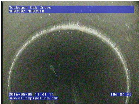
GM3676_29b5a4f6-782c-44a4-b604-e6dda5d2d56c_20160505_114251_000.jpg, 00:17:44, 106.83 Joint Offset Medium
