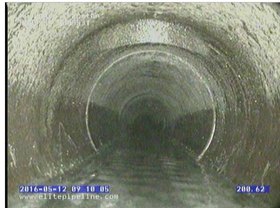
GM3700_d760bc2d-7738-420b-a21c-0e3d9fae79d8_20160512_091123_807.jpg, 00:13:23, 200.60 Tap Factory Made at 12 o'clock, 6inch dim, within 8 inch
