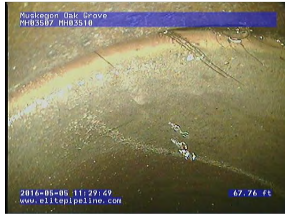
GM3676_29b5a4f6-782c-44a4-b604-e6dda5d2d56c_20160505_113126_184.jpg, 00:09:52, 67.05 Infiltration Runner at 1 o'clock, within 8 inch
