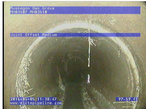
GM3676_29b5a4f6-782c-44a4-b604-e6dda5d2d56c_20160505_114024_426.jpg, 00:15:44, 97.58 Joint Offset Medium
