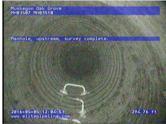
GM3676_29b5a4f6-782c-44a4-b604-e6dda5d2d56c_20160505_120629_923.jpg, 00:37:24, 294.75 Manhole, upstream, survey complete.
