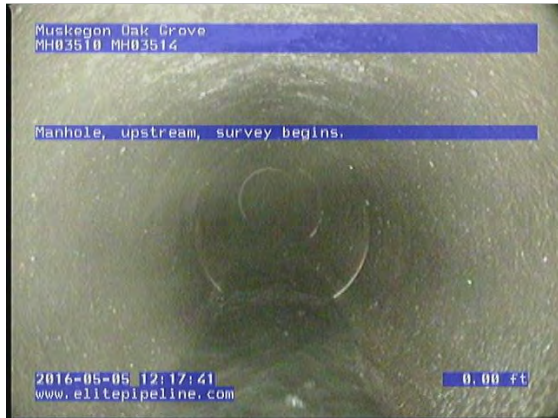
GM3683_ed2824f5-d3e3-4757-88d6-d4208adc31ee_20160505_121917_971.jpg,00:00:26,0.00 Manhole, upstream, survey begins.
