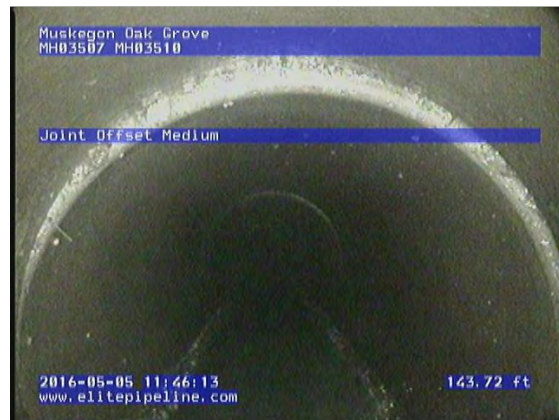
GM3676_29b5a4f6-782c-44a4-b604-e6dda5d2d56c_20160505_114750_654.jpg, 00:21:47, 143.71 Joint Offset Medium
