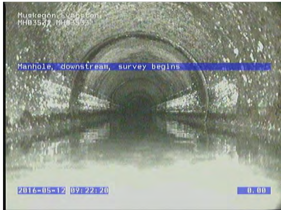
GM3701_62c62d3f-fa26-4182-aa9d-10e119c32db3_20160512_092339_488.jpg, 00:00:20, 0.00 Manhole, downstream, survey begins
