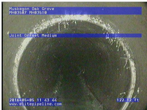
GM3676_29b5a4f6-782c-44a4-b604-e6dda5d2d56c_20160505_114521_356.jpg, 00:19:34, 122.11 Joint Offset Medium
