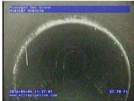
GM3676_29b5a4f6-782c-44a4-b604-e6dda5d2d56c_20160505_112838_179.jpg, 00:08:04, 57.68 Joint Offset Medium
