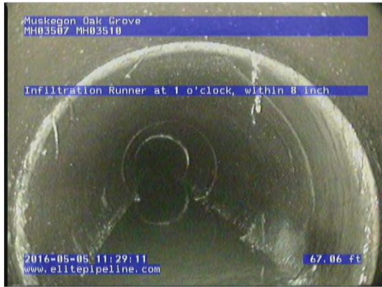
GM3676_29b5a4f6-782c-44a4-b604-e6dda5d2d56c_20160505_113047_904.jpg, 00:09:52, 67.05 Infiltration Runner at 1 o'clock, within 8 inch
