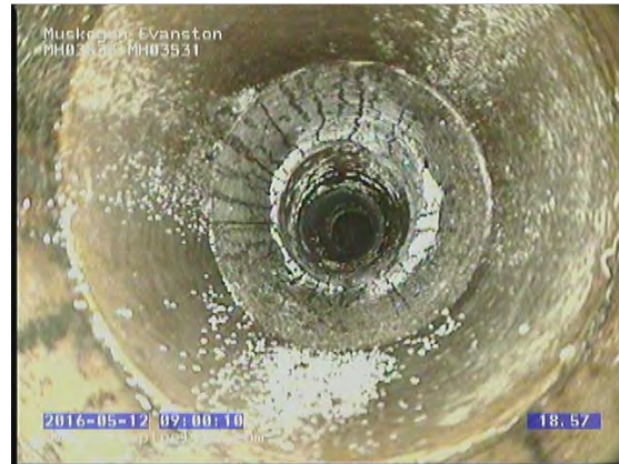
GM3700_d760bc2d-7738-420b-a21c-0e3d9fae79d8_20160512_090129_333.jpg, 00:03:48, 16.89 Tap Factory Made Active at 12 o'clock, 6inch dim, within 8 inch
