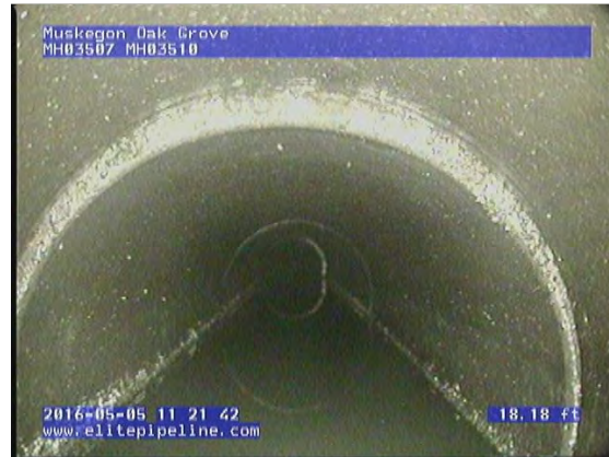
GM3676_29b5a4f6-782c-44a4-b604-e6dda5d2d56c_20160505_112319_350.jpg, 00:03:45, 18.18 Joint Offset Medium
