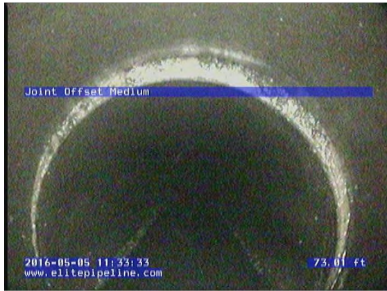
GM3676_29b5a4f6-782c-44a4-b604-e6dda5d2d56c_20160505_113510_230.jpg, 00:11:59, 73.01 Joint Offset Medium
