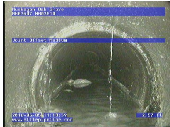
GM3676_29b5a4f6-782c-44a4-b604-e6dda5d2d56c_20160505_112016_223.jpg, 00:01:26, 2.57 Joint Offset Medium
