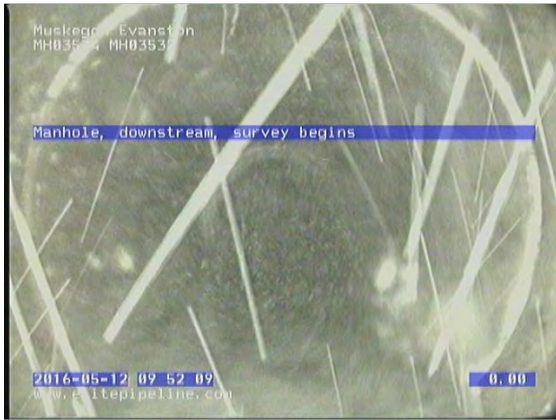
GM3702_bffedebf-8262-4dd8-8638-19abd94e99a5_20160512_095328_625.jpg, 00:00:20, 0.00 Manhole, downstream, survey begins
