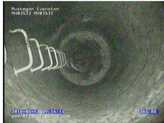
GM3700_d760bc2d-7738-420b-a21c-0e3d9fae79d8_20160512_091733_376.jpg, 00:18:21, 264.87 Manhole, upstream, survey complete.
