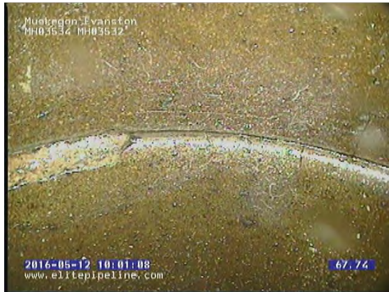
GM3702_bffedebf-8262-4dd8-8638-19abd94e99a5_20160512_100227_024.jpg, 00:07:52, 67.73 Infiltration Dripper at 11 o'clock, within 8 inch
