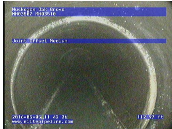
GM3676_29b5a4f6-782c-44a4-b604-e6dda5d2d56c_20160505_114402_747.jpg, 00:18:34, 112.97 Joint Offset Medium
