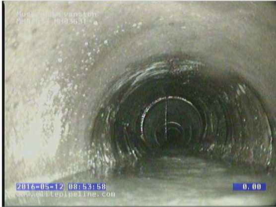
GM3700_d760bc2d-7738-420b-a21c-0e3d9fae79d8_20160512_085517_579.jpg, 00:00:19, 0.00 Manhole, downstream, survey begins
