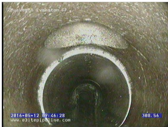
GM3701_62c62d3f-fa26-4182-aa9d-10e119c32db3_20160512_094747_063.jpg, 00:22:07, 308.55 Tap Factory Made Capped at 12 o'clock, 6inch dim, within 8 inch
