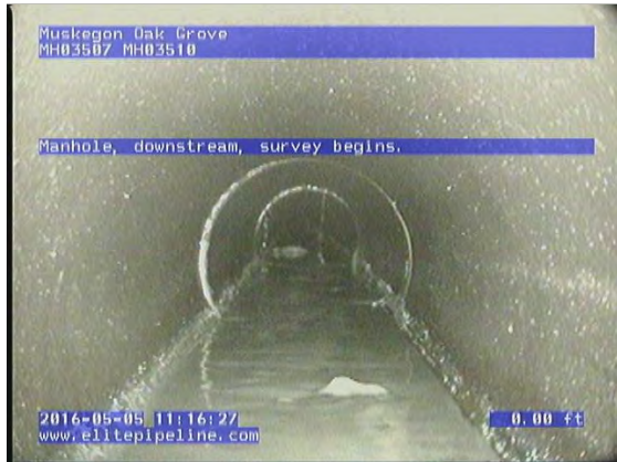
GM3676_29b5a4f6-782c-44a4-b604-e6dda5d2d56c_20160505_111804_486.jpg, 00:00:25, 0.00 Manhole, downstream, survey begins.
