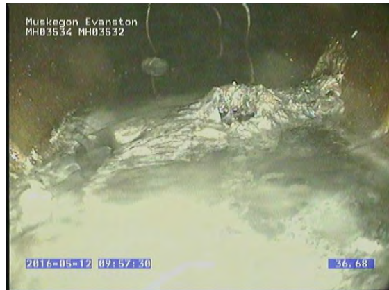
GM3702_bffedebf-8262-4dd8-8638-19abd94e99a5_20160512_095849_203.jpg, 00:04:43, 36.68 Deposits Settled Other, 10% of cross sectional area from 5 o'clock to 7 o'clock, Debris
